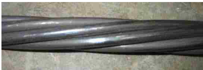
Figure 4.1 Strand exterior after exposure to 500°F (260°C)
