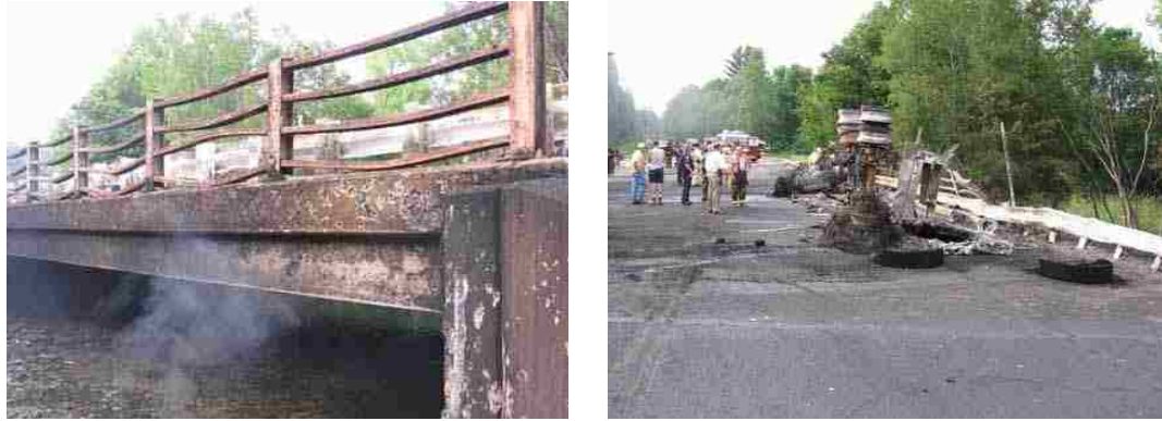
Figure 6.1 Aftermath of the bridge fire along U.S. Route 7 Bridge near Ridgefield, Connecticut (FHWA, 2007)
