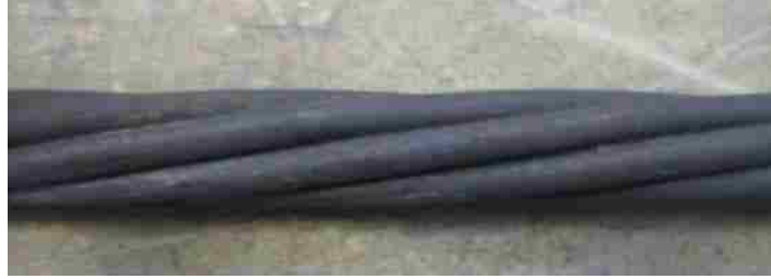
Figure 4.3 Strand exterior after exposure to 1000°F (538°F)
